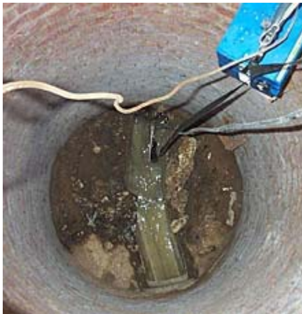
Figure 4. Open-channel flowmeters are called for when the liquid of interest is not closely confined or pressurized. The Model 2150 area-velocity meter shown here monitoring flow at the bottom of a manhole does not require a weir or flume, although many such flowmeters do. (Photo courtesy of Isco, Inc. )
