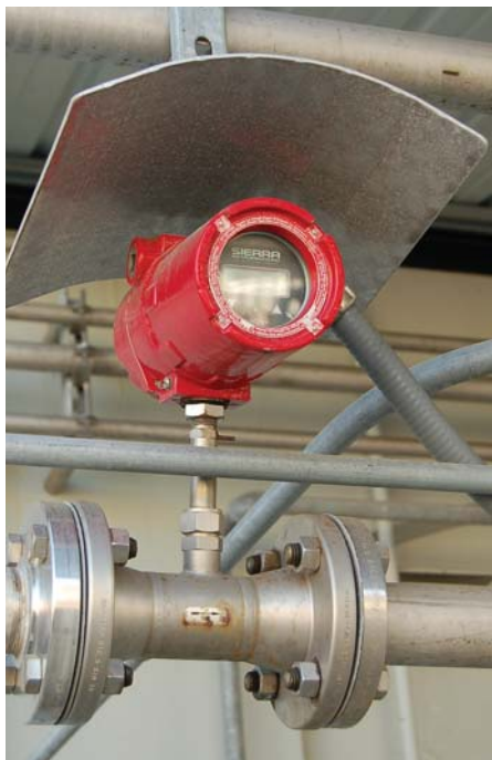
Here an immersible thermal mass flowmeter is used in a bio gas application. Photo courtesy of Sierra Instruments Inc. ( www.sierrainstruments.com ).
