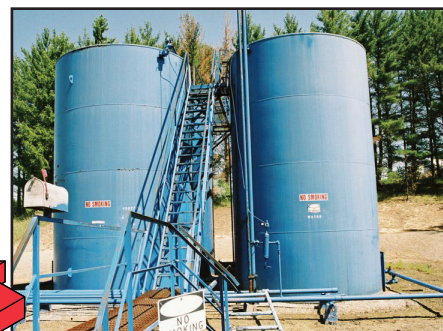
When oil is removed from a well, it is typically in a mixture with gas and water. Once the oil is separated out, it is often held in storage tanks until it is transferred by pipeline or by truck to a refinery.
