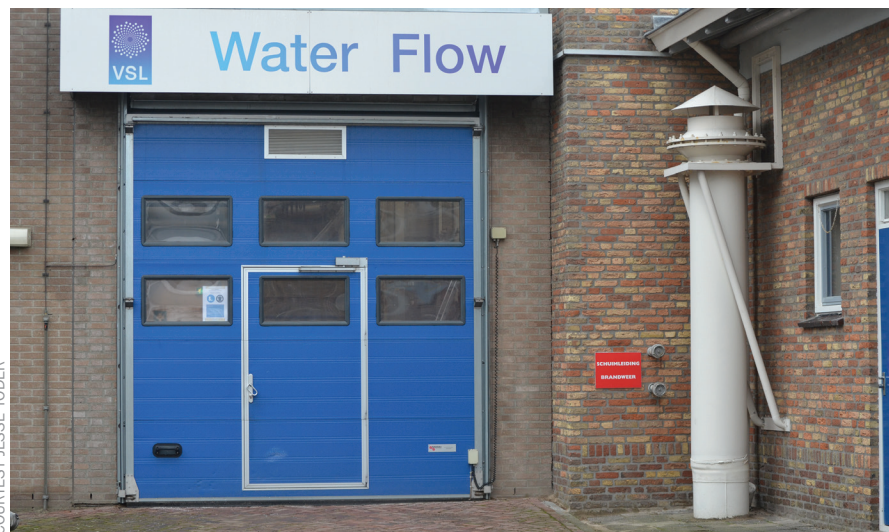
VSL's liquid flowmeter calibration facility in Dordrecht, the Netherlands.
