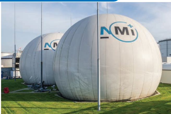
Natural gas storage balloons at an NMI Euroloop gas flow calibration facility.
