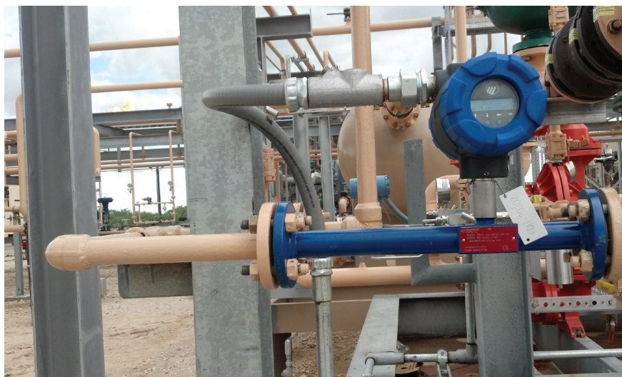
Here a Magnetrol flow-body (spool-piece) type inline sensor measures natural gas for an exploration and production company.
