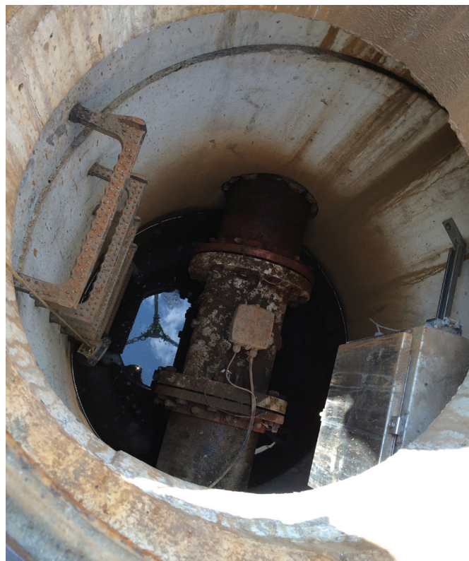
Battery-operated capability is enabling magnetic flowmeter technology to be employed in various new applications where direct wiring is difficult, such as the water distribution monitoring system pictured here.
