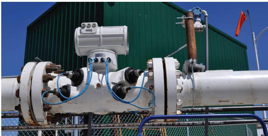
Inline ultrasonic meters have two or more transducers embedded into the flowmeter (sensor tube) body. They are installed by cutting into a pipe and having either wafer or flange style fittings. (Photo courtesy of Flow Research)
