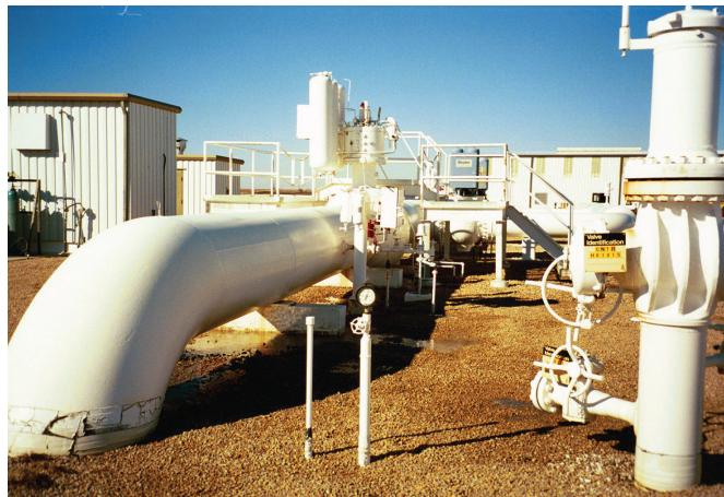
A 42-inch natural gas supply pipeline at CEESI's natural gas custody transfer station in Iowa.
