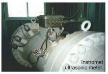
transducer travels through the flow stream, its frequency shifts in proportion to the mean velocity of the fluid. The reflected signal is detected by a receiver, which measures its frequency. The meter calculates flow by comparing the transmitted and reflected frequencies.
