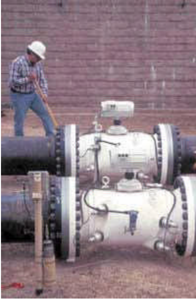
FIG. 3: The publication of AGA-9, specifying the criteria for the use of ultrasonic flowmeters in natural gas custody transfer applications, has opened up new opportunities for these flowmeters. Shown is a 20-in. Senior Sonic ultrasonic flowmeter by Daniel.
